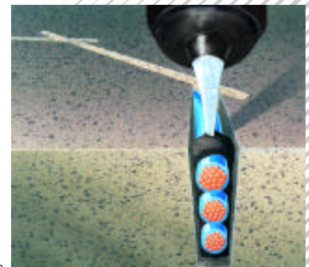
4. Fill sawcut with 3M ® Detector Loop Sealant.
